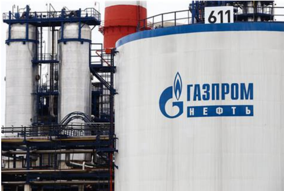
Figure 5. catalytic cracking unit
