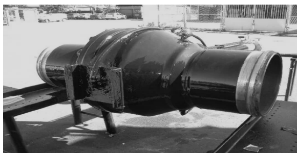
Fig. 2. Application of the "Protegol" Anti-Corrosion Coating by Germany's TIB Chemicals Company
