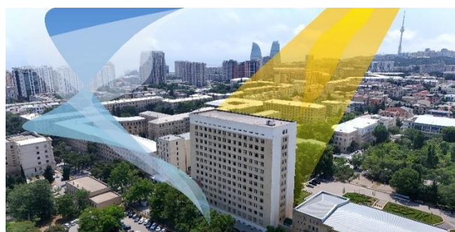
Figure 3. Drone View Illustrating the Impact of Solar Radiation and Wind on the Second Educational Building
